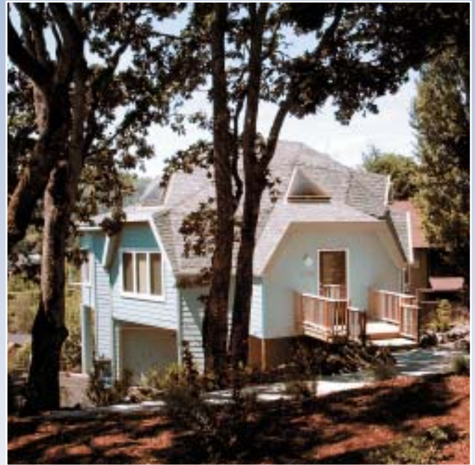
Three bedroom, three bath home. 35 foot diameter dome on five-foot riser-wall on lower level with tuck under garage. From 2000 to 2400 square feet, including 400 square foot garage.
