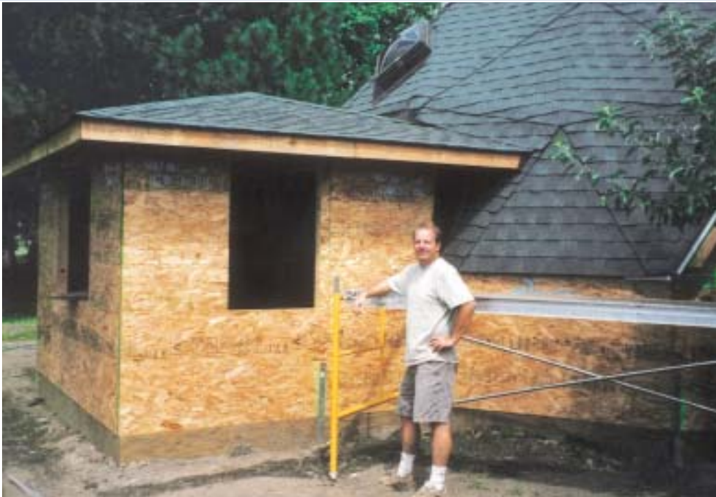
Roger Boothe, Dome Raising Supervisor, raised a 30 foot diameter dome on a four-foot riser-wall with rectangular shaped PVR in a day with an all volunteer crew. Roofers arrived the next day to install the roofing in four days.
