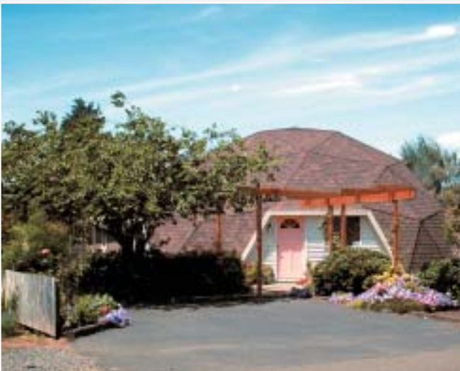
45 and 50 foot diameter domes are popular and the best home values available today. The loft in these 3/8 sphere domes are bedroom(s), bath or study. When a lower level for garage, recreation, storage, and living space is planned, a 3,300-5,000 square-foot home is possible.
