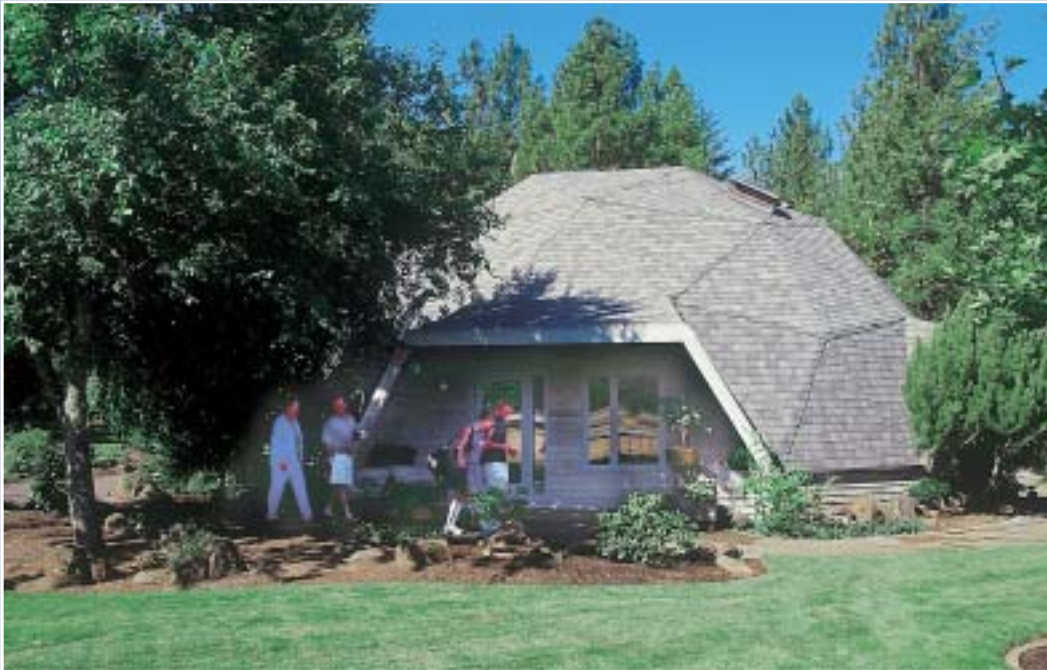
Linda, Roger, Carie and Wills enjoy Oregon Dome Living. 50 foot diameter dome on two-foot riser-wall with four-foot porch extensions.
